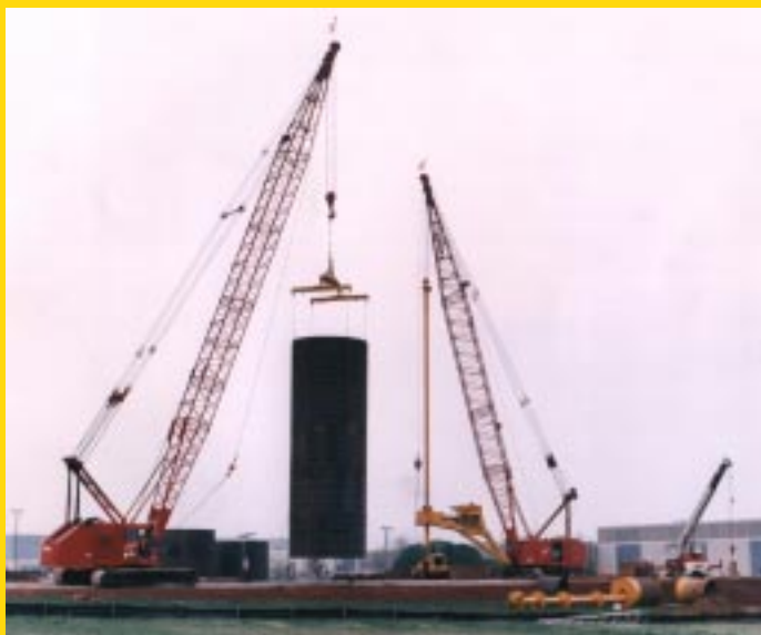
INSTALLATION OF 17.5-FOOT DIAMETER, 50-FOOT LONG CASING.
