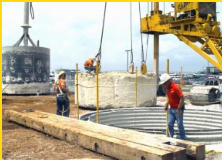
15.5-FOOT DIAMETER AIR CORE BARREL AND 15.5-FOOT DIAMETER LIMESTONE CORE.
