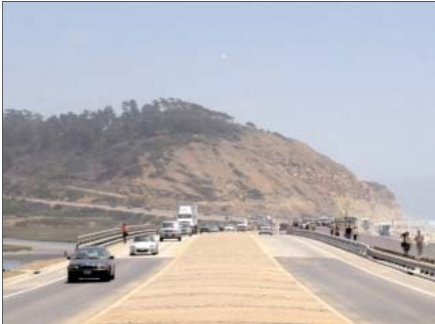
Both pedestrian and vehicle traffic move easily over the new structure.
