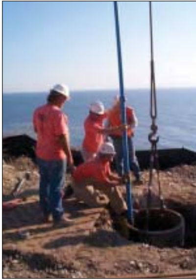
Crew installs inclinometer.
