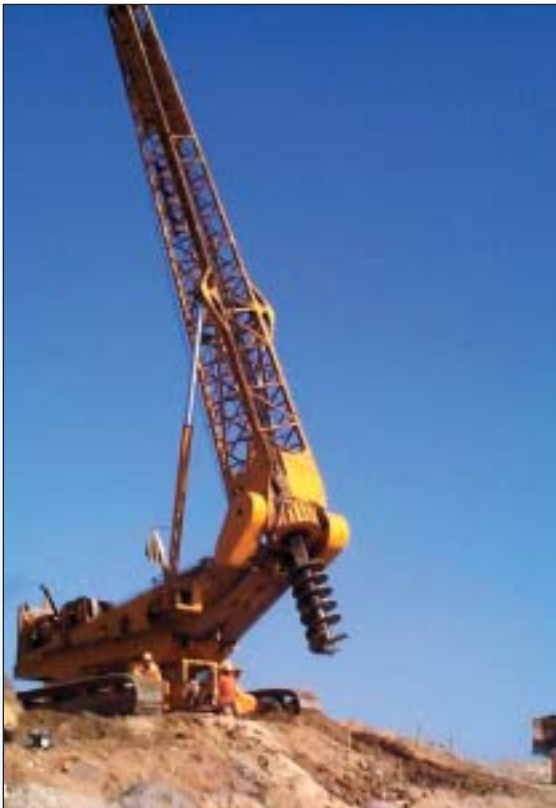
"Big Stan Moving" to a new shear pin location.
