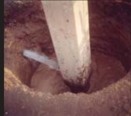
Denver area practice of "mudding the hole"
