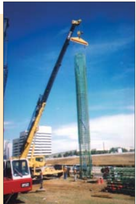
The reinforcing cages were formidable
