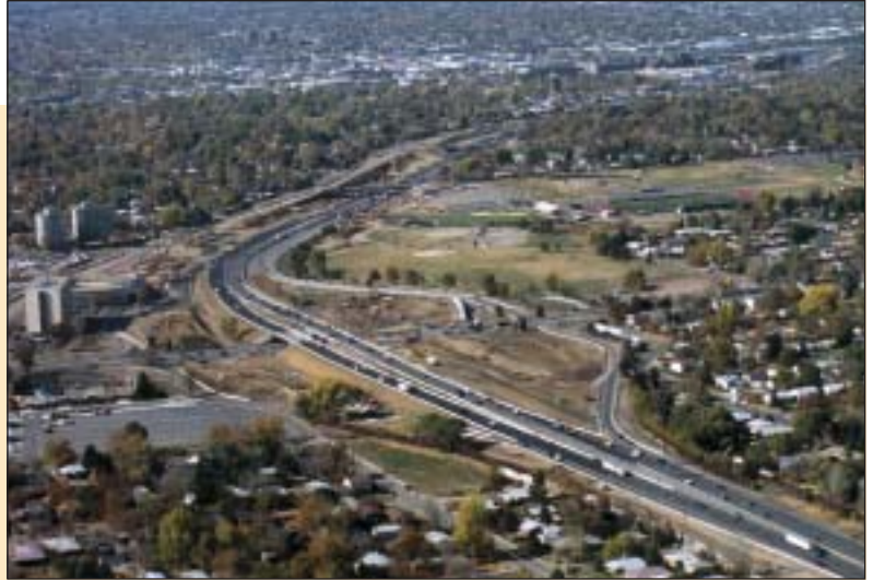
T-REX, I-25 Improvement cuts north-south right through Denver.
