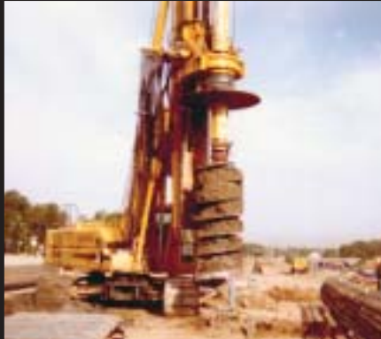
The rig and the soil
