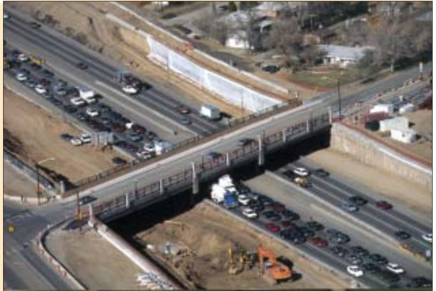
The bottlenecks to be alleviated by widening the roadway. Note drilled shaft soldier wall under construction.
